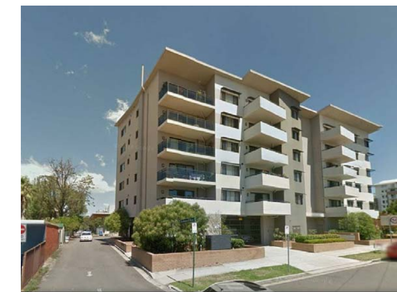
A. Adjoining Building: 16-18 Lachlan Street
