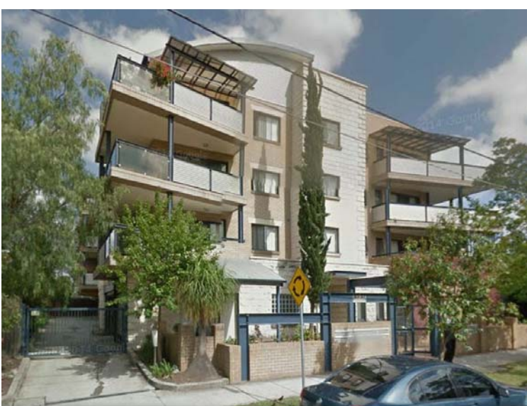
B. Adjoining Building: 25-27 Goulburn Street
